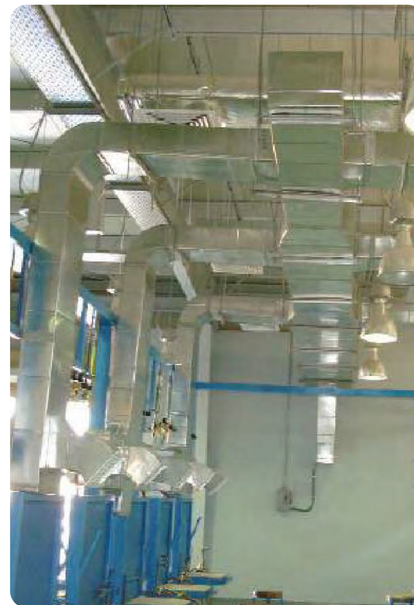
HVAC Work at Royal Vocational Training Center Al-Riyadh
