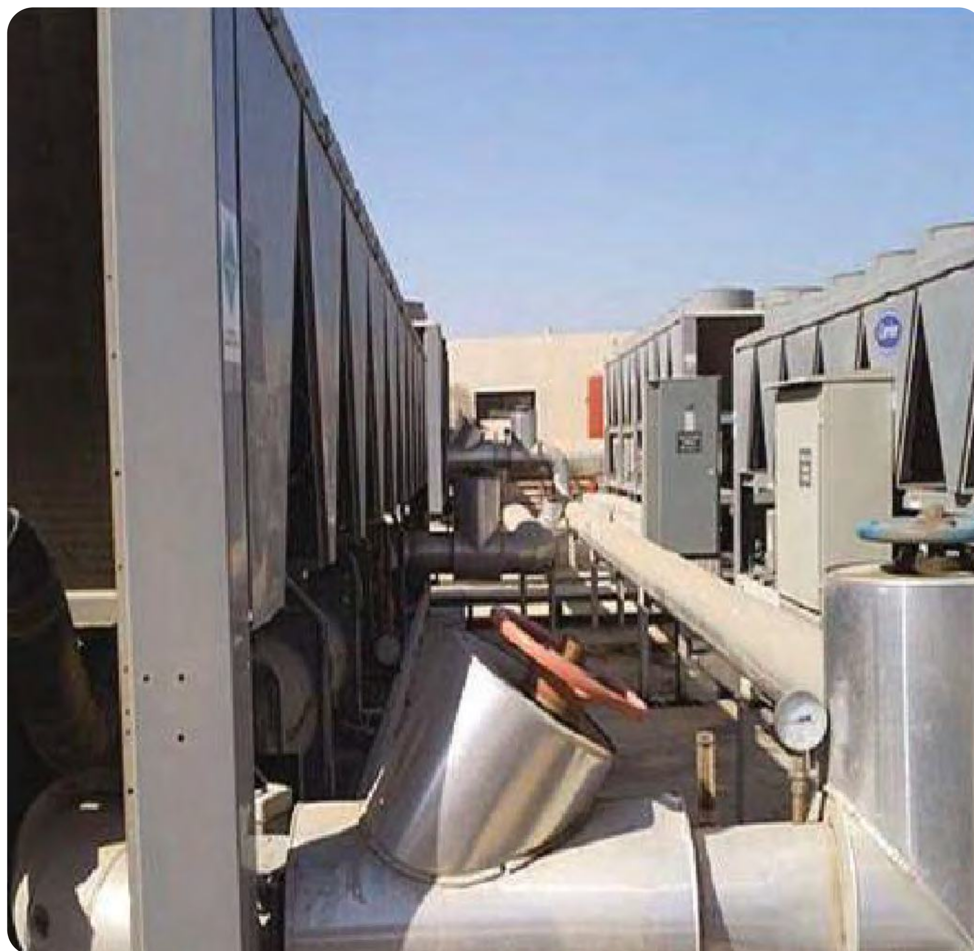
Chiller Works at King Abdulaziz University at Jeddah
